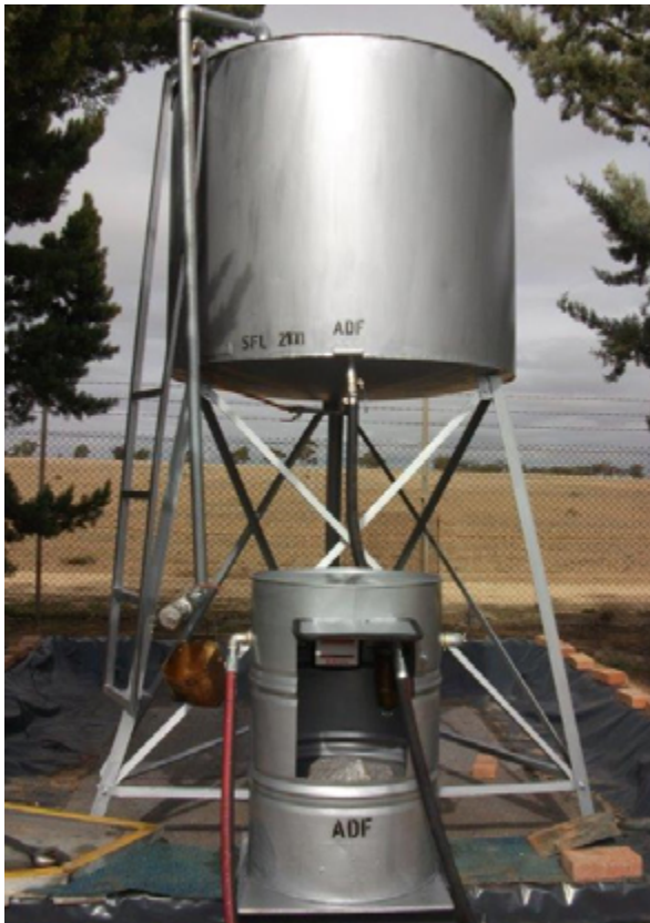
Figure 7 Elevated tank with hose connection point at ground level Photo courtesy Ben Wade
