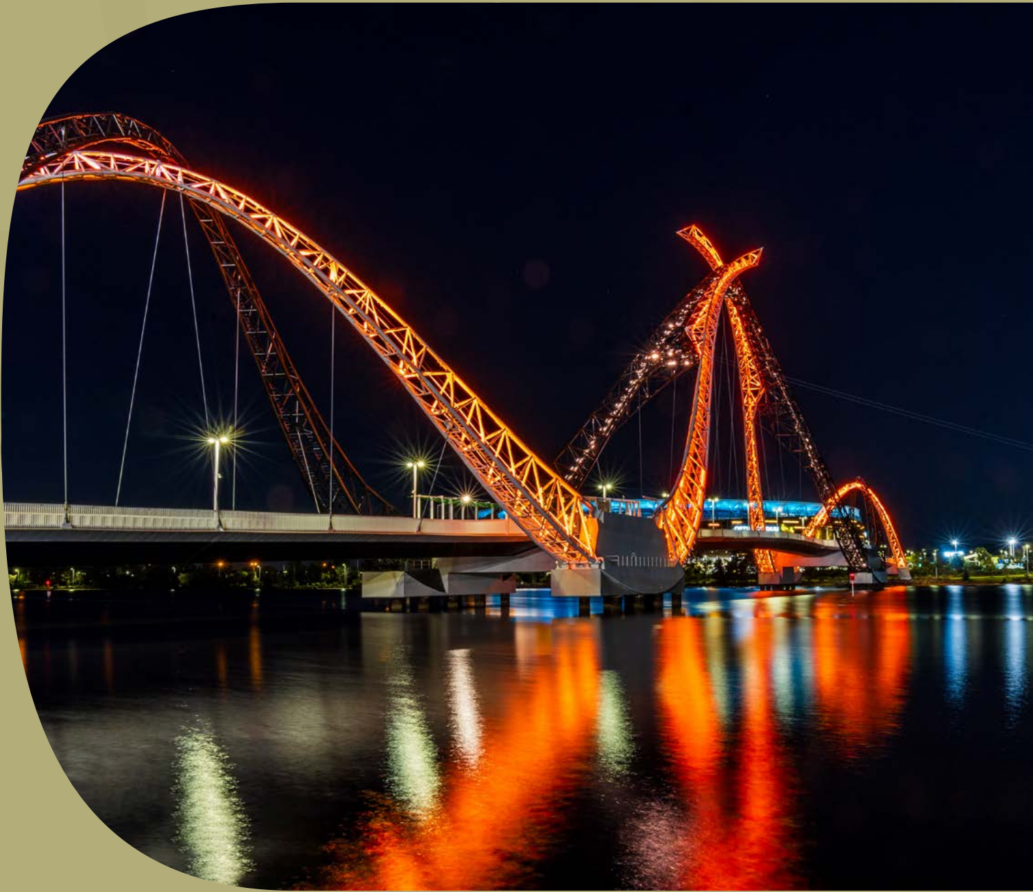
Matagarup Bridge was lit up for Safe Work Month 2023.
