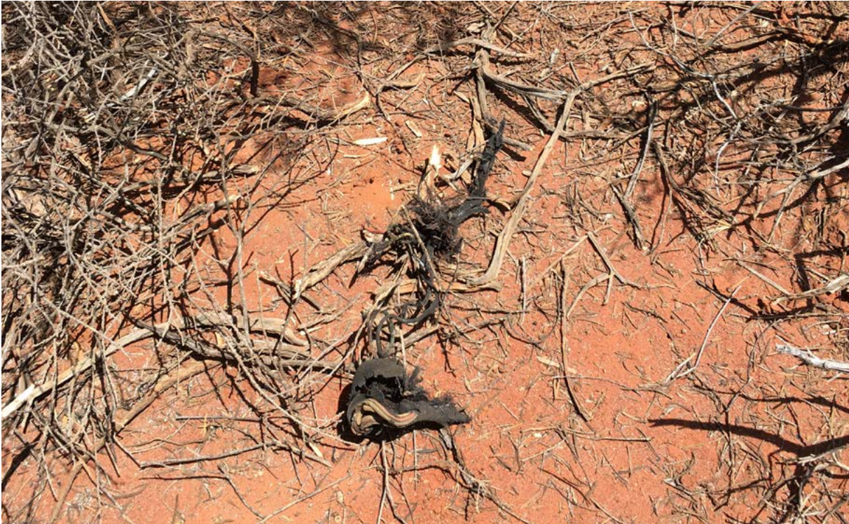
Figure 5.31 Fire damaged electrical cabling 132 m east-south-east of the epicentre of the explosion
