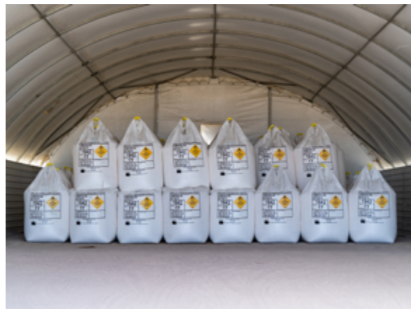
Figure 3.2 A modern, light-weight, cost effective dome structure for dedicated, stand-alone IBC storage
