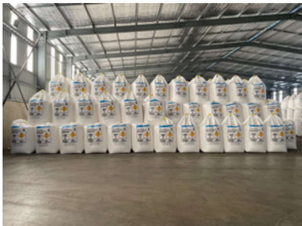
Figure 3.1 A 9,000 tonne, high security, steel and concrete building for dedicated, stand-alone IBC storage
