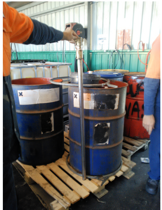
Figure 4 Metal (conductive) pipe for transfer of flammable liquids sufficiently long enough to avoid splashing and generation of static electricity
