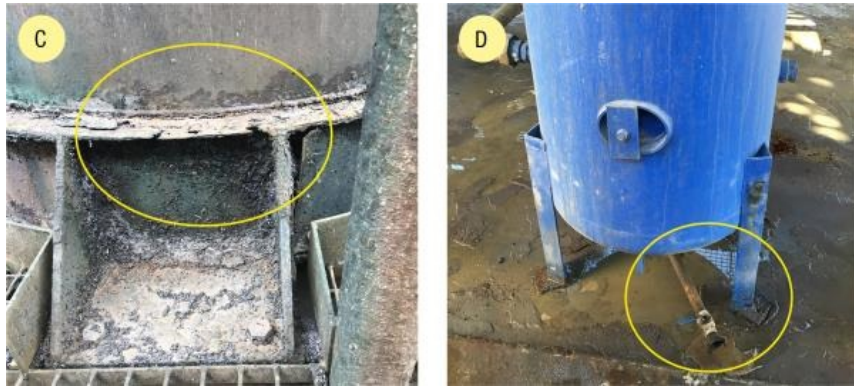
Pressure vessel supports. A. Unanchored vessel containing refrigerated argon gas. B. Air receiver leg anchored to grating only. C. Severe corrosion of a support bracket to an acid elution column (condition of shell unknown). D. Air receiver not bolted down and connection point corroding.
