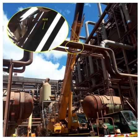
While slewing a crane, the operator focused on the load and congested surroundings. A spotter instructed the crane operator to stop when he saw the boom was close to the acid line. By the time the crane operator ceased the movement, the boom had contacted and fractured the fibreglass acid line, resulting in acid spraying onto the crane.
