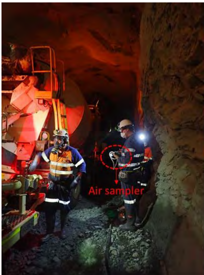
Figure 10: Air sampling during the Shotcreting activity.
